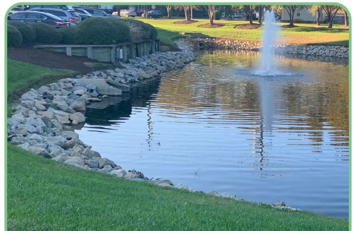
Typical Stormwater Pond
