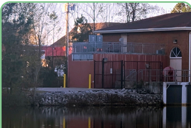
Typical Stormwater Pump Station
